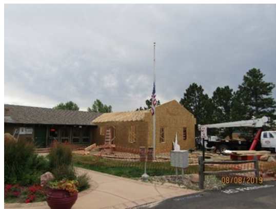
Exterior Walls & Roof Trusses
