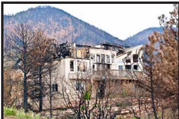
Mt. Shadows home destroyed because of lack of defensible space.
